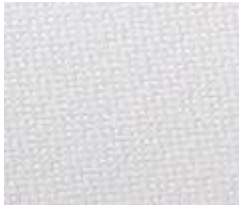
Ceiling sheathing Gainage plafond
